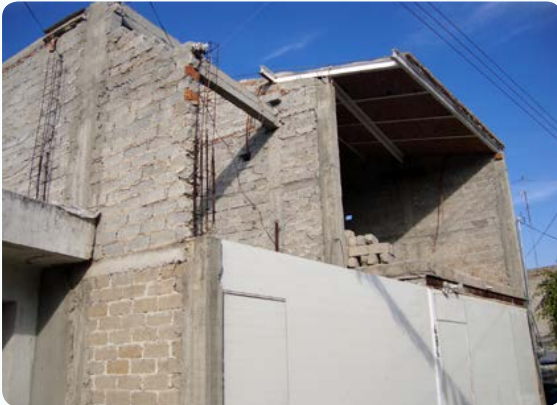
A socio's home under construction.
