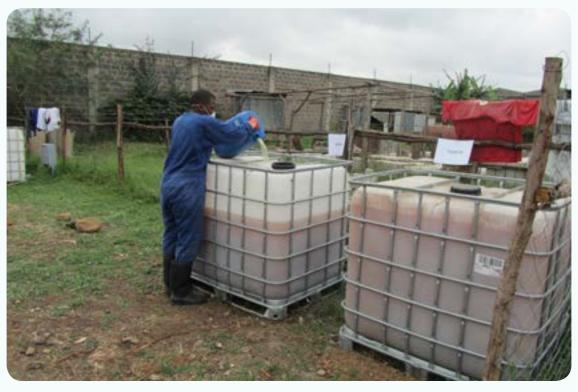
Urine holding tanks. No waste, solid or liquid ever goes into the natural equipment. There is no chance for waste to leach into the soil and for the high water table to flood the toilets during the rainy season (as stated on Sanergy's website).
