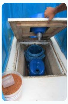
The urine diverting mechanism is under the FLT toilet plate.
